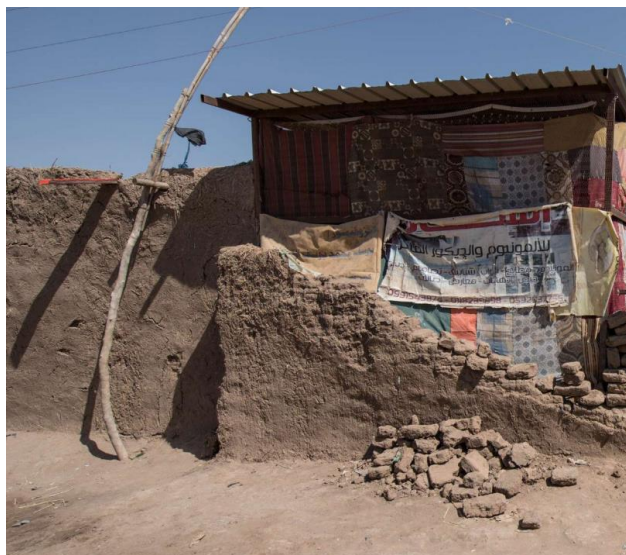
Image 1: Showing a house in Mayo partially damaged after the rains season. (The Italian Agency for Development Cooperation AICS - Khartoum office, 2021)
