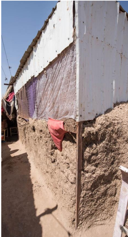
Figure 8: Picture showing the variety of materials used in building, one builds on top of another as each follows a collapse event. Source: Taken by Stefano Rosso, November 2020, edited by author.
