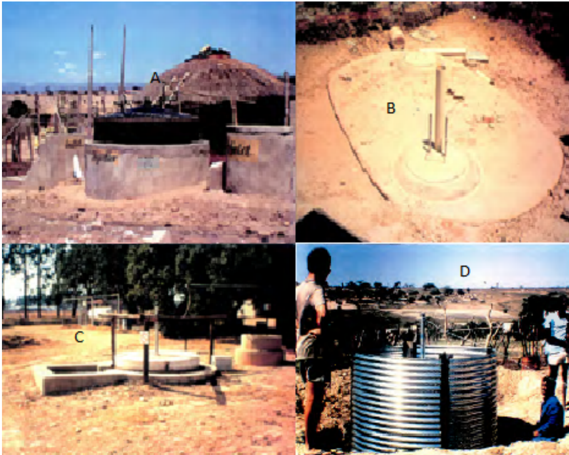
Figure 4: A: The floating-drum biogas plant that was built at the homestead of the Mathabela family in Gazankulu. B: The biogas digester that was installed at the Mzimhlophe Secondary School in KwaNdebele. C: The floating-drum biogas plant that was installed at the University of Pretoria's experimental farm. D: The galvanised iron mould used to build the Ferro cement digester at the homestead of the Mathabela family (Thom 1994).
