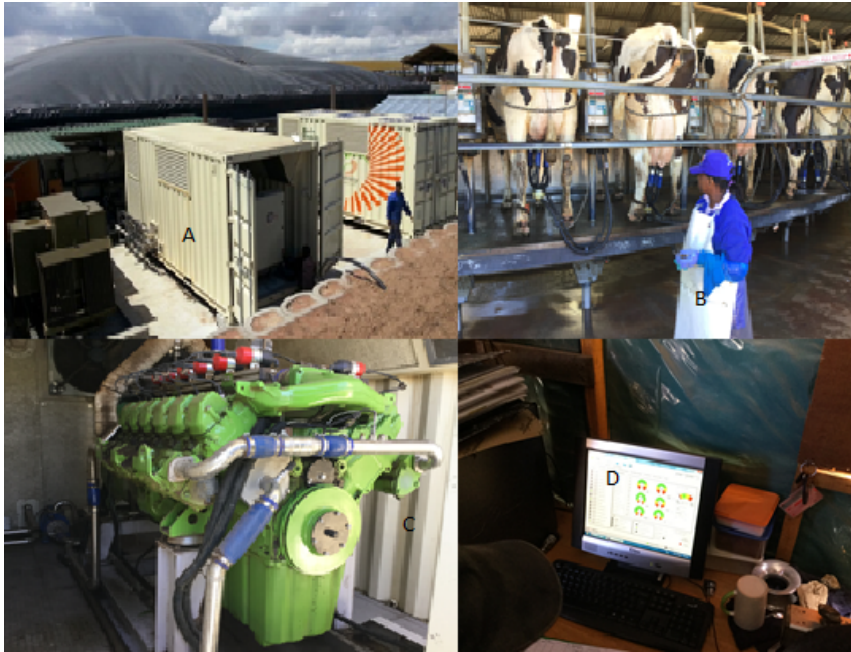
Figure 6: A-Lagoon digester adjacent to generators, B- Dairy cows, C-Gas engine, D- Control room (Basson 2016).
