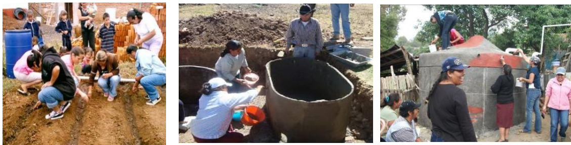
Figure 3. Installation process of appropriate technologies.
